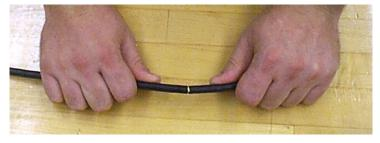
Figure 4 – Flex the cable to separate the cable jacket.
