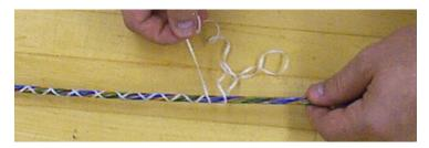
Figure 21 – Unwrap the binder threads from the buffer tubes.
