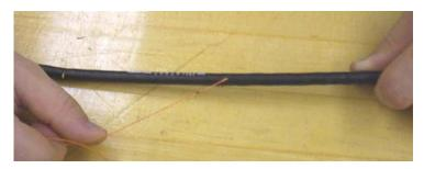
Figure 7 – Pull the ripcord through the outer jacket.
