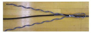
Figure 12 – Wrap the dead-end onto the cable.
