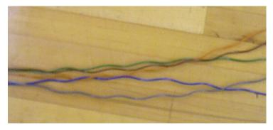
Figure 22 – Separate the buffer tubes from the central strength member.
