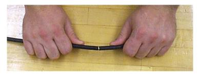
Figure 17 – Flex the cable to separate the jacket.
