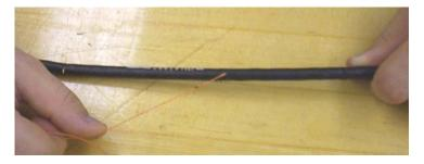
Figure 19 – Pull the ripcord through the outer jacket.
