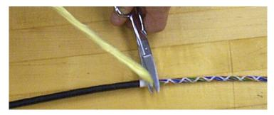
Figure 20 – Cut the strength members to length as required.
